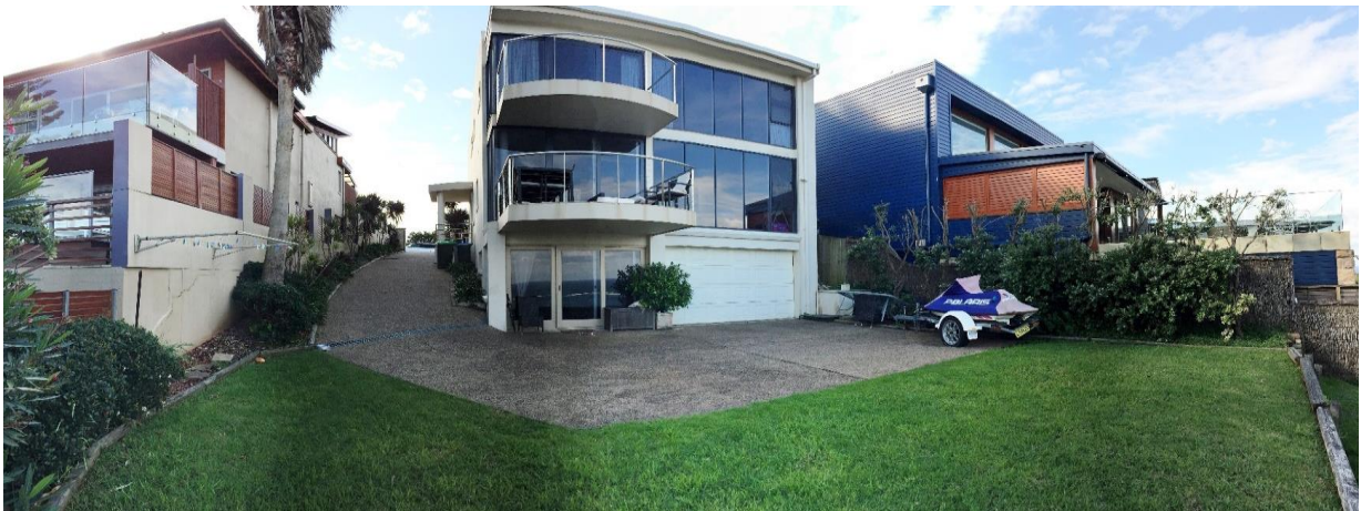
Figure 1: Photo of existing rear elevation of primary dwelling on subject site & the greater rearward alignment of both adjoining properties
