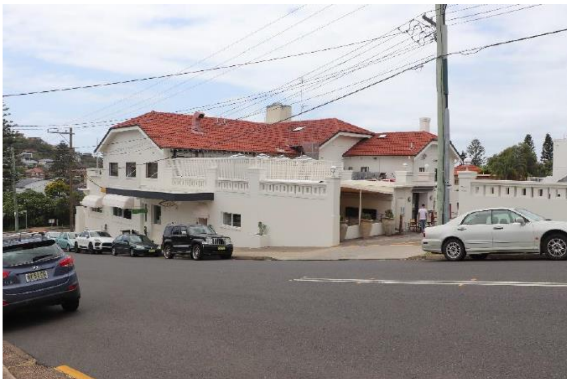
Figure 10 – Comparison images showing the increased roof level in the south-eastern corner of the existing hotel premises and relatively minor additional height and scale
