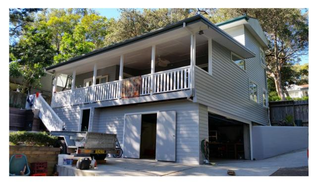
NEW WEATHERBOARD CLADDING TO MATCH EXISTING INCLUDING WALL COLOUR TIMBER FASCIAS AND TRIM - WHITE TO MATCH EXISTING ALUMINIUM WINDOWS – WHITE TO MATCH EXISTING NEW COLORBOND ROOFING AND GUTTERS TO MATCH EXISTING METAL ROOFING AT REAR INCLUDING COLOUR – WOODLAND GREY
