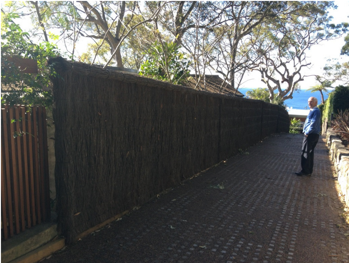
Figure 2: Section of fencing along northern side of access handle
