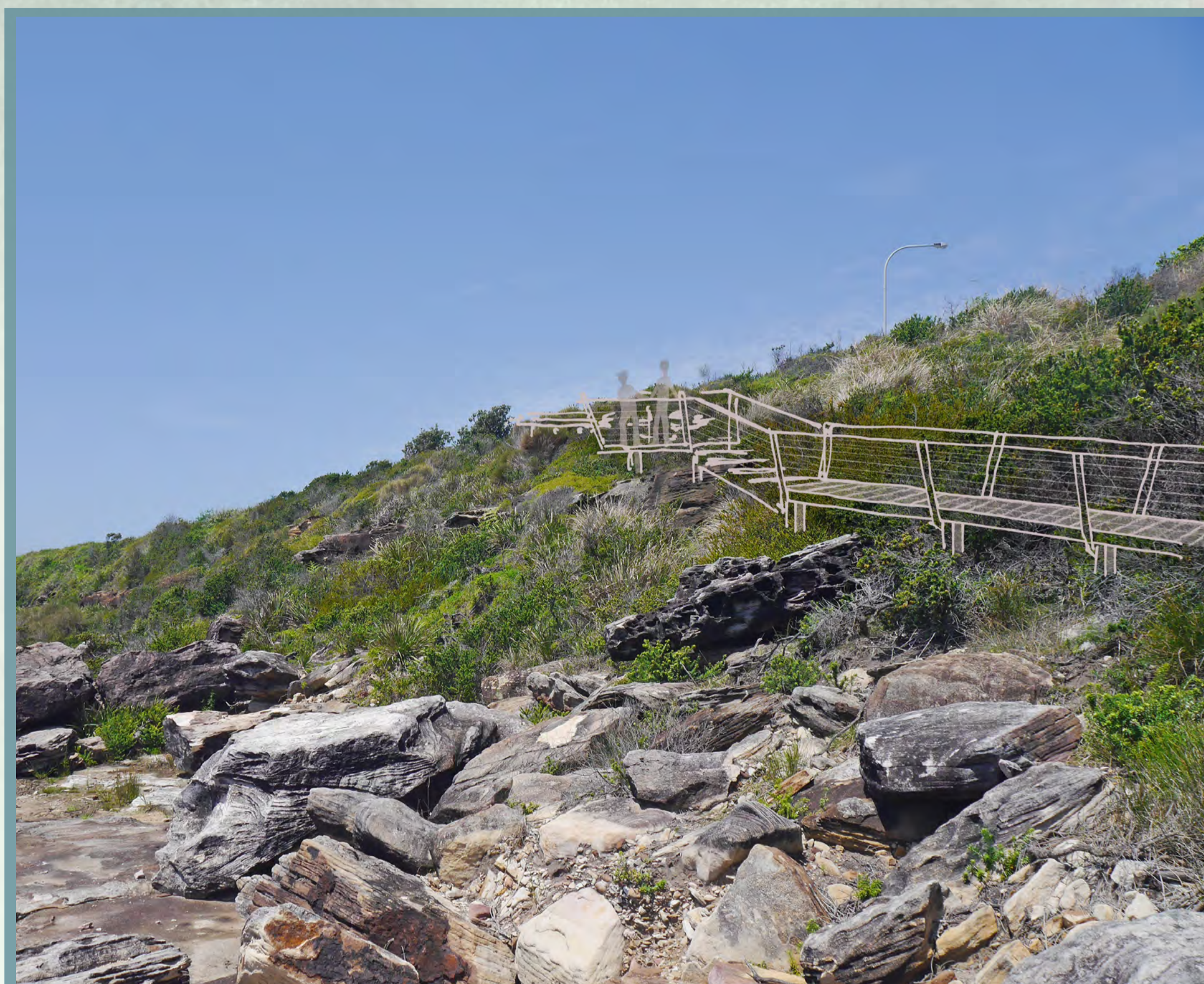
2 SKETCH CONCEPT OF ELEVATED BOARDWALK THROUGH VEGETATION Sensitively designed elevated boardwalk is situated above and clear of the existing native vegetation supported on posts attached to the rock below, resulting in minimal impact to indigenous vegetation and the visual character of the area. The proposed alignment will traverse at a gentle gradient through an area of younger vegetation to avoid damaging mature native species in nearby steep coastal banks.
