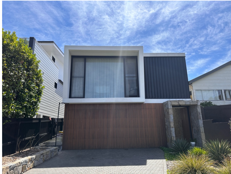
View of Site from Austin Avenue
