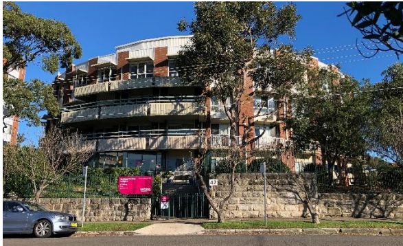
Figure 10: View of existing hostel at the northern part of the site, looking directly west from Birkley Road (Source: Google Streetview)
