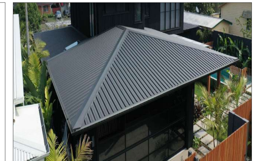
3. COLORBOND MONUMENT METAL ROOF
