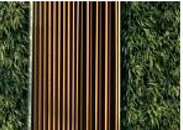
S5-Vertical Battens over Glazed Wall
