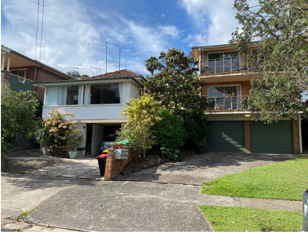
Photograph of the site and the adjoining three (3) storey RFB to the west – 17 Baltic Street
