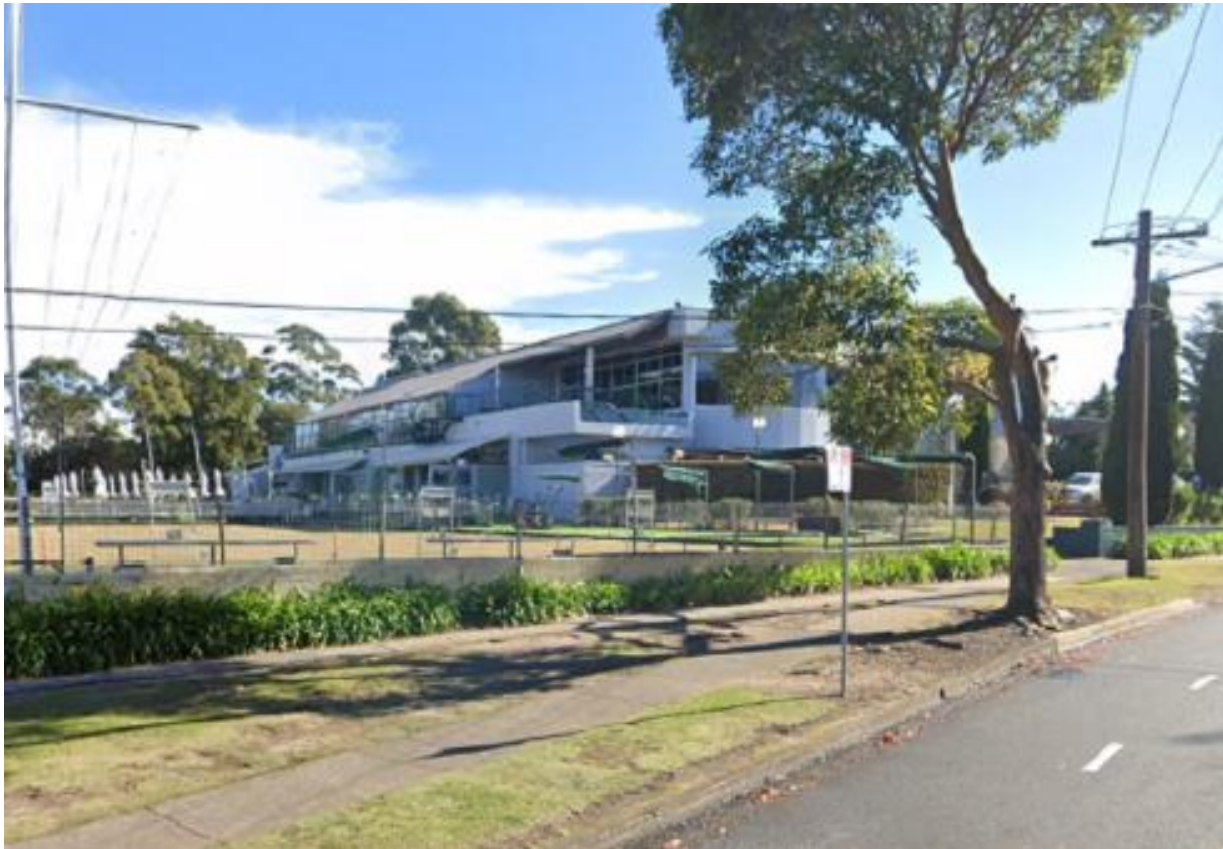
Figure 2 - Subject property as viewed from Melwood Avenue
