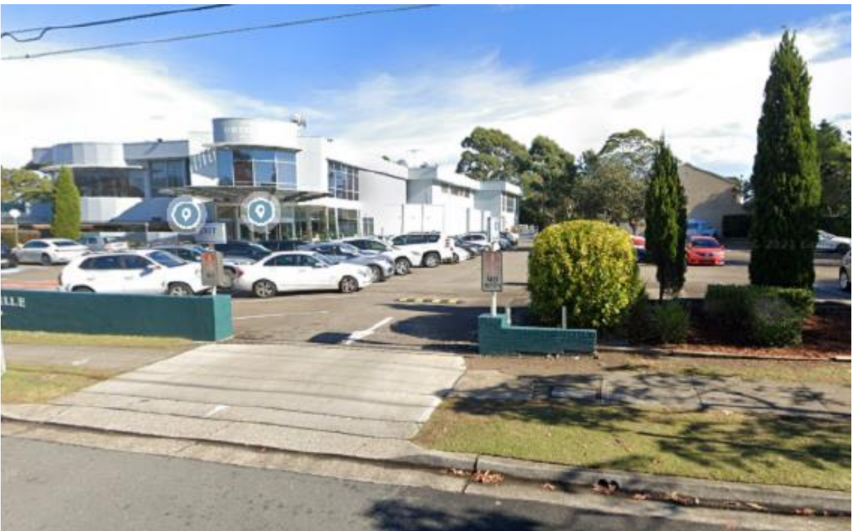
Figure 4 – Northern end of subject property as viewed Melwood Avenue
