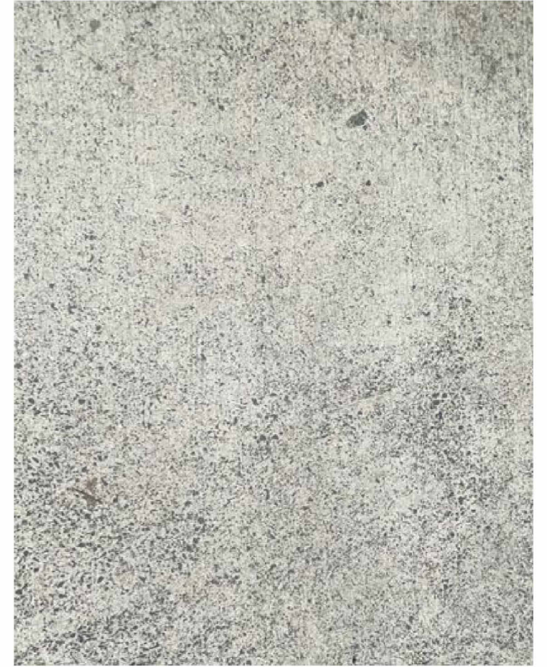
FLOOR FINISH - CAR SPACE CONCRETE
