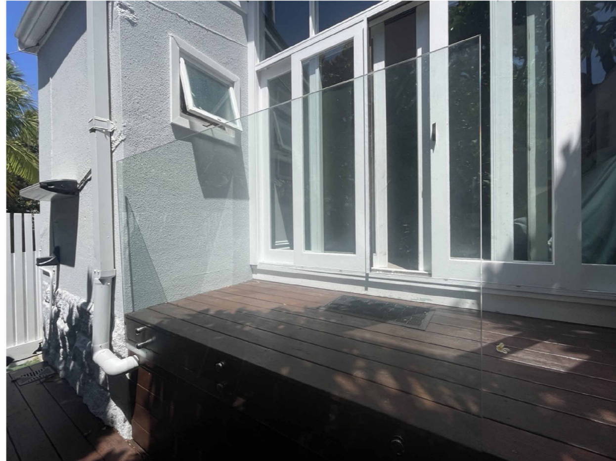
BALUSTRADE GLASS (TO MATCH EXISTING AT REAR)
