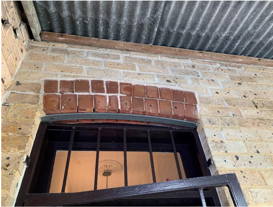
Repaired arch entry above door and top highlight. Note dislodgement of top corner brickwork and sliding away from bull nose verandah rafter.
