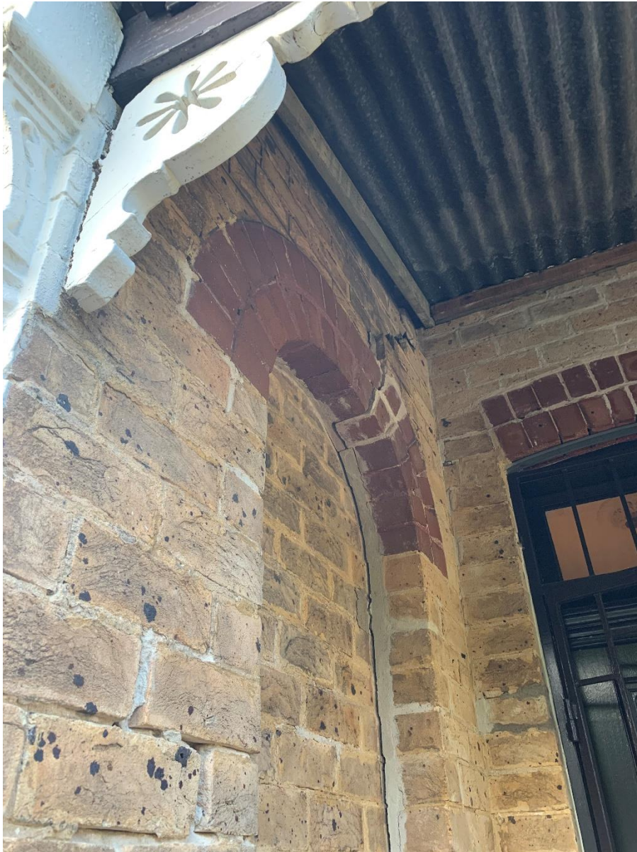
Unsuccessful mortar repair work. Note thickness and out of plumb wall.
