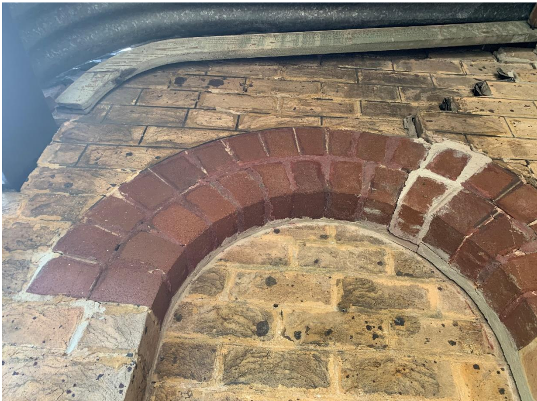
Displaced arch (inside of common blade common fire wall). Note movement from roof rafter at bull nose and attempted unsuccessful repairs to mask displacement. Cracking and movement evident.
