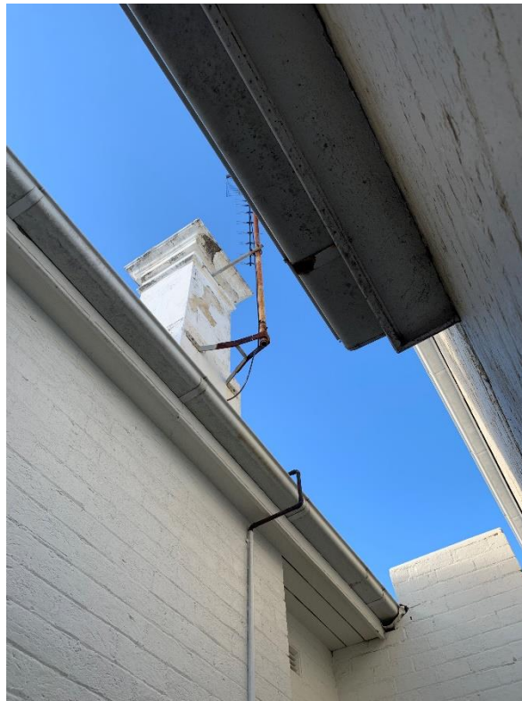
Rear second chimney. Note side walls have been painted and is to be reclaimed and reconstructed.
