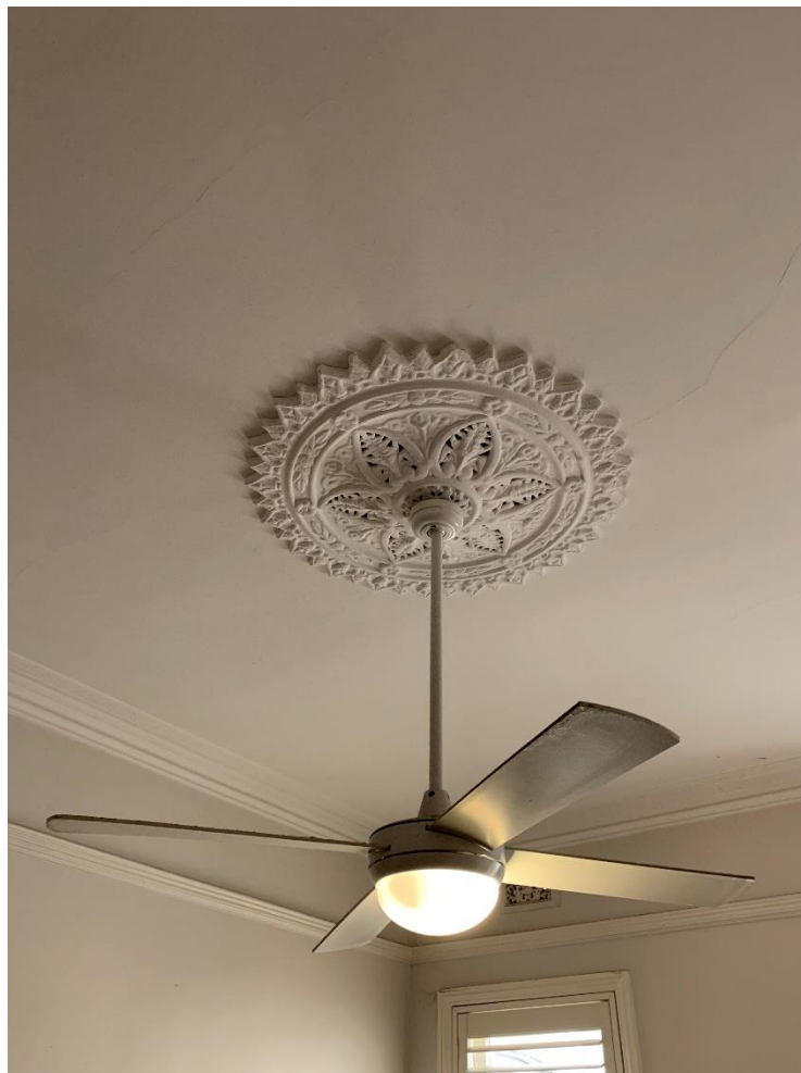
Period ceiling, cornices, picture rail, architraves and ceiling rose.
