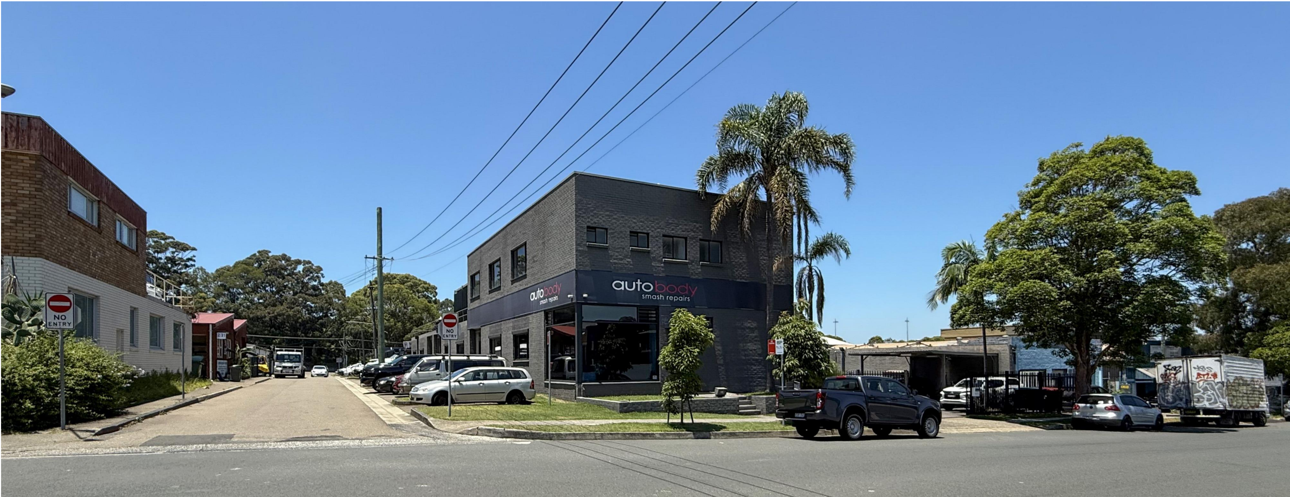
1 - VIEW FROM CORNER OF CARTER ROAD & WEST STREET - EXISTING
