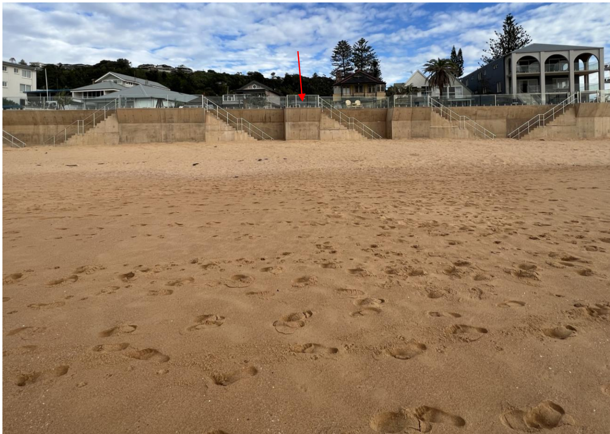
Figure 1: View of subject property (at arrow) from Collaroy Beach, facing west, on 3 June 2022
