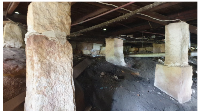
Figure 13 – Sandstone columns beneath house
