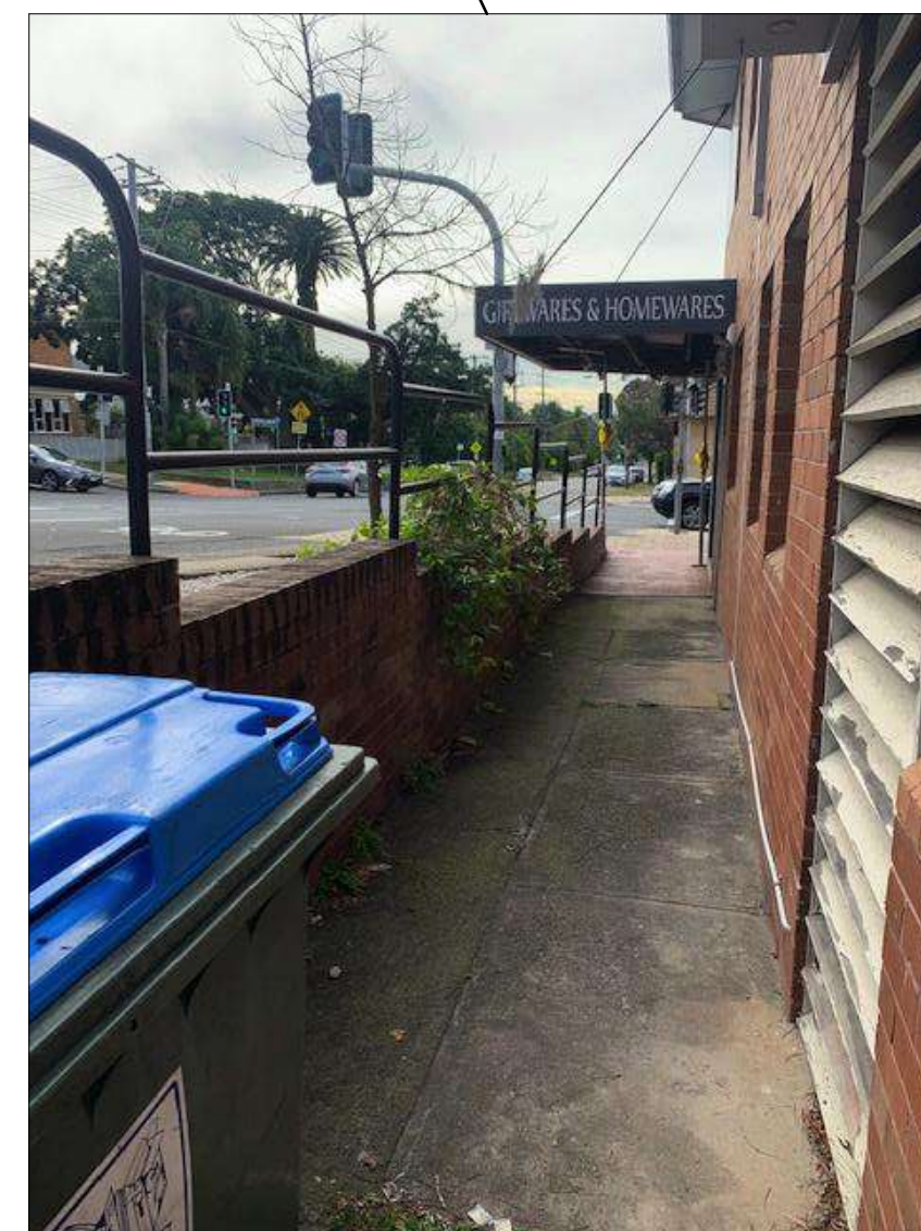
EXISTING RETAINING WALL ALONG OLIVER STREET TO ACCOMMODATE THE SLOPE OF THE ROAD. SIMILAR APPROACH USED WITH THE PROPOSED SCHEME FOR THE OUTDOOR SEATING AREA
