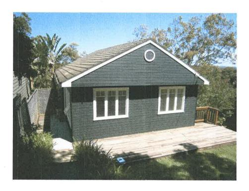
**Weatherboard - Studio** – Weathertex Primelok Shadowood smooth 170mm weatherboards. Colour to match the existing house
