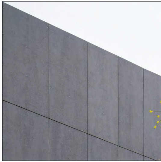
FC: FIBRE CEMENT SHEET CLADDING EQUITONE 'SOFT GREY' OR EQUIVALENT
