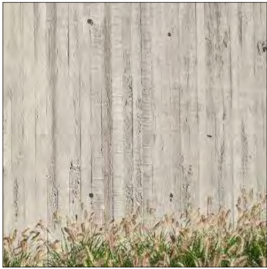
CON: CONCRETE OFF-FORM CONCRETE WITH TEXTURED FINISH
