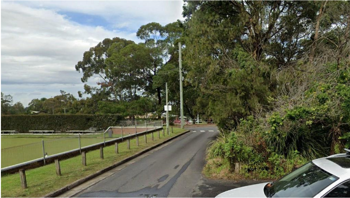
Figure 6: Existing Laneway View towards the South
