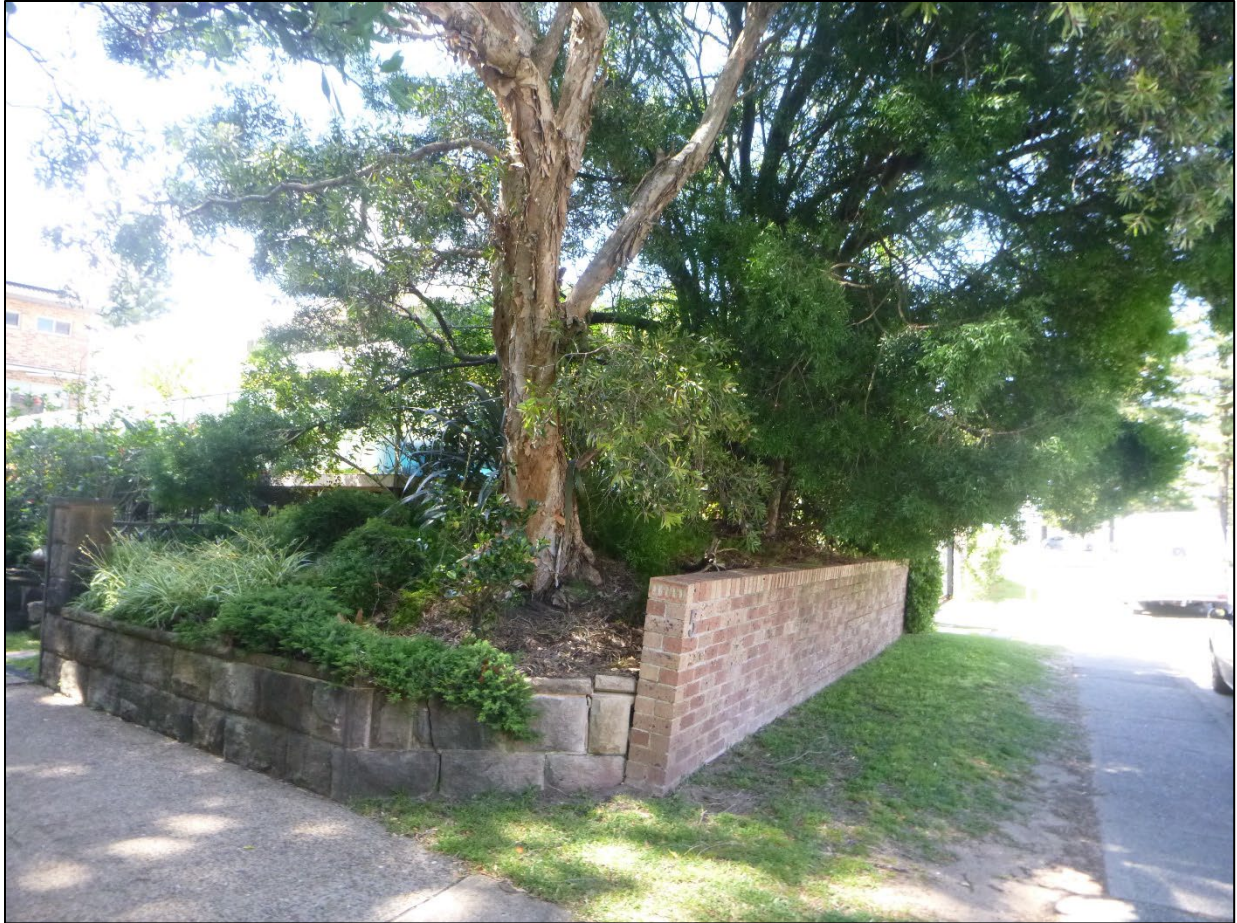
Photo B: Wall displacement and cracking is influenced by the root plate expansion of Trees 3 and 4.
