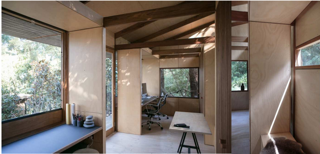
INTERNALS: PLY LINING HILIGHTS AND EXPOSED HARDWOOD FRAMING/HARDWOOD INTERNAL DOOR FRAMES.
