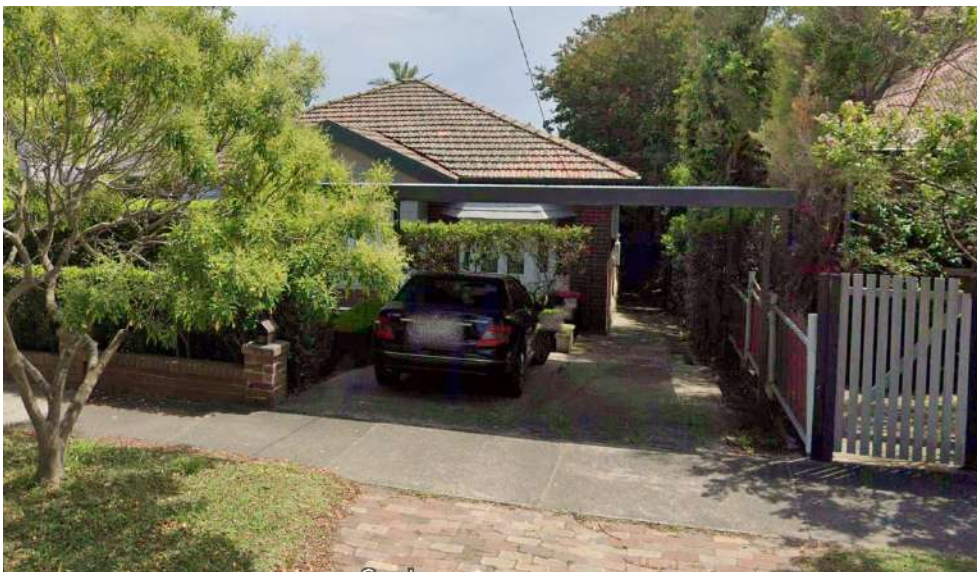
Figure 12. Carport at 6 Jamieson Avenue
