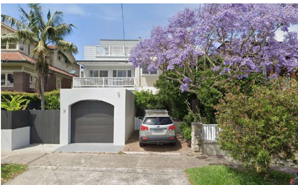
Figure 15. Garage at No. 7 Jamieson Avenue.
