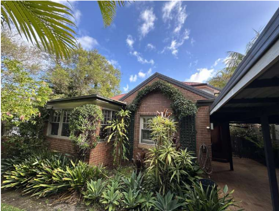
Figure 6. The dwelling façade, looking north.
