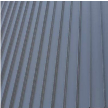
METAL SHEET ROOFING-over new terrace
