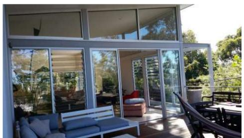
NEW ALUMINIUM HILITE WINDOW TO NORTH ELEVATION OF FIRST FLOOR LIVING ROOM ADDITION TO MATCH EXISTING WINDOWS
