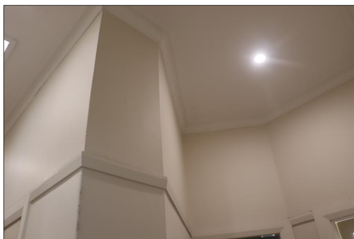
Figure 38: Typical coved cornice detail and picture rail.
