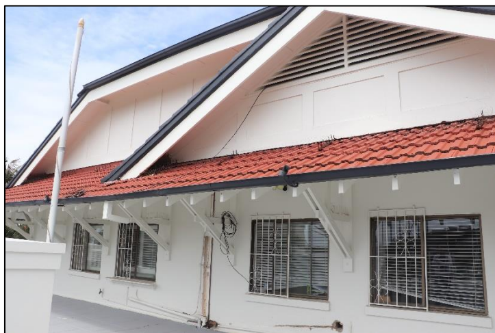
Figure 20: Detail of tiled verandah roof and sliding aluminium framed windows.
