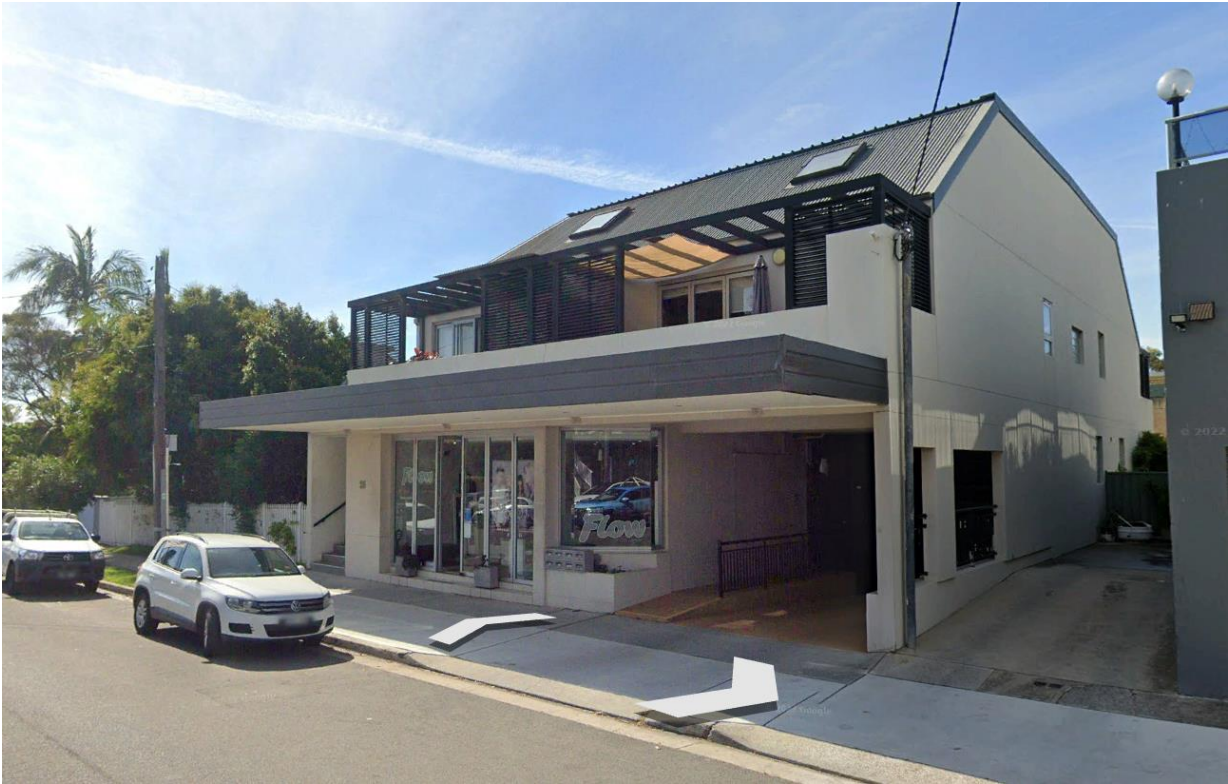
Figure 5: View towards 26 Ocean Grove occupied by a two storey mixed-use building
