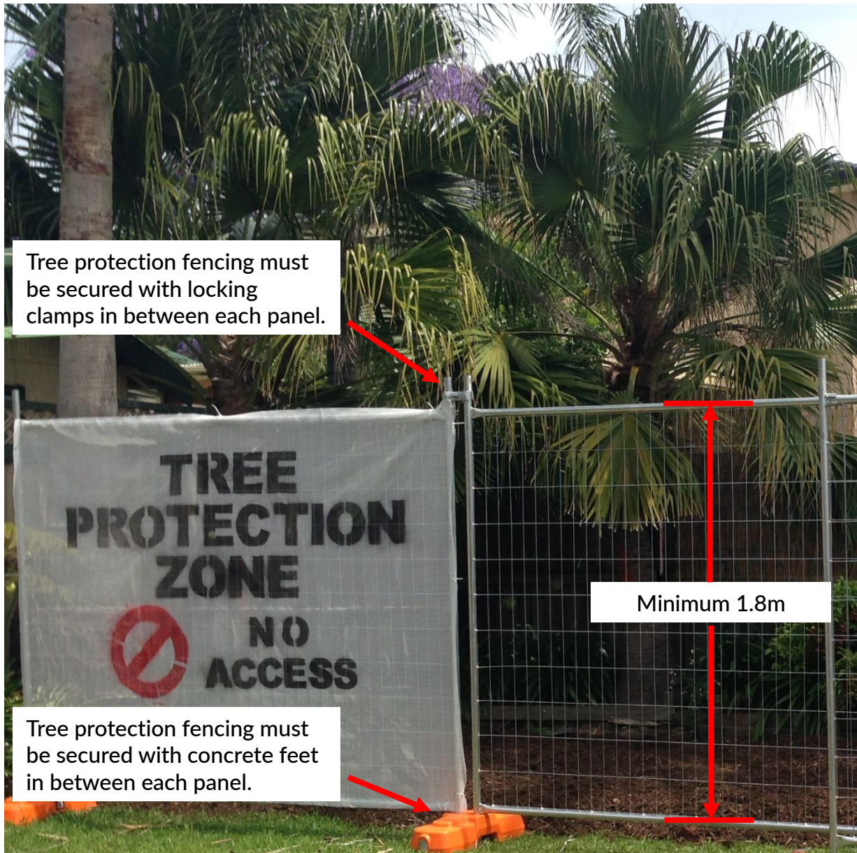
An Example of Temporary Fencing
