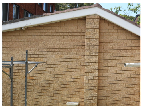
1. FACE BRICK - TO MATCH EXISTING AUSTRAL BRICK - EVERYDAYLIFE RANGE - RETREAT OR SIM.
