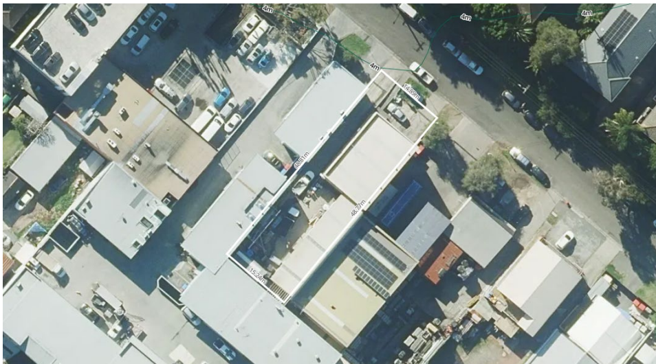
Figure 2: Site aerial (Source: EMC report)
