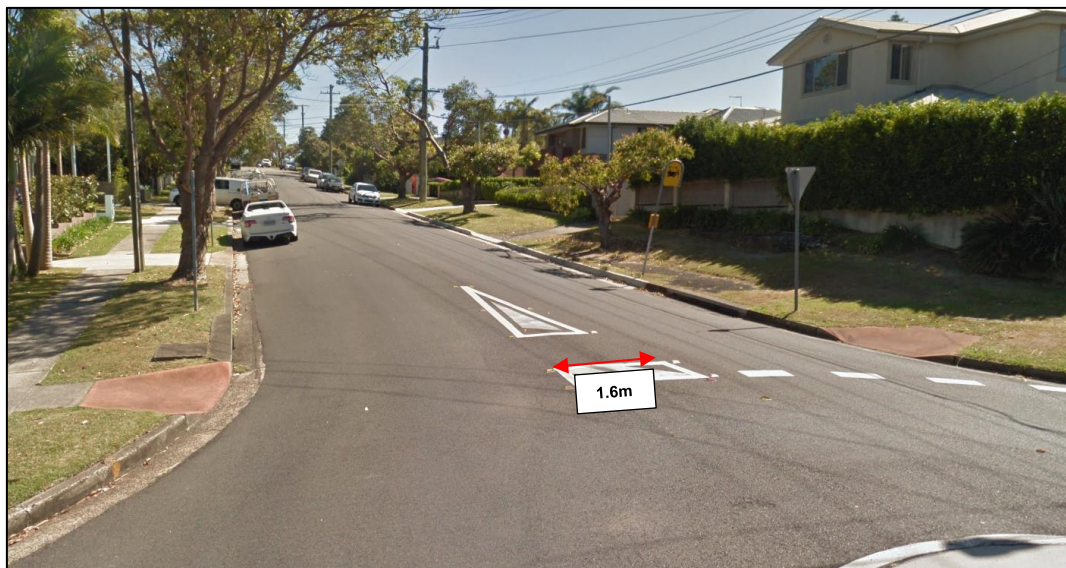
FIGURE 1: EXISTING ROUNDABOUT SPLITTER ISLAND
