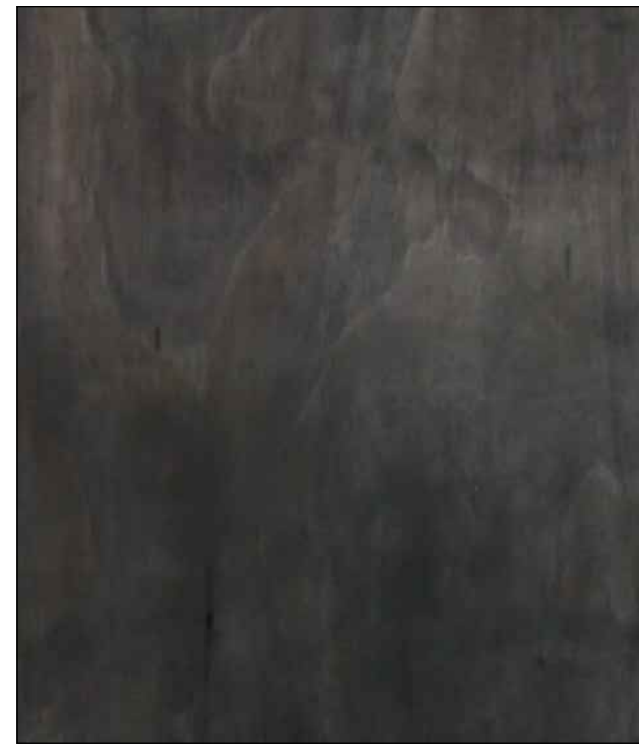
3 BLACKENED STEEL FRAMING
