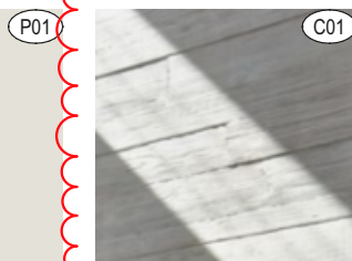
OFF FORM CONCRETE
