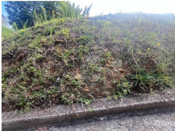
Photo 3: Extremely weathered shale bedrock outcropping in the driveway cutting
