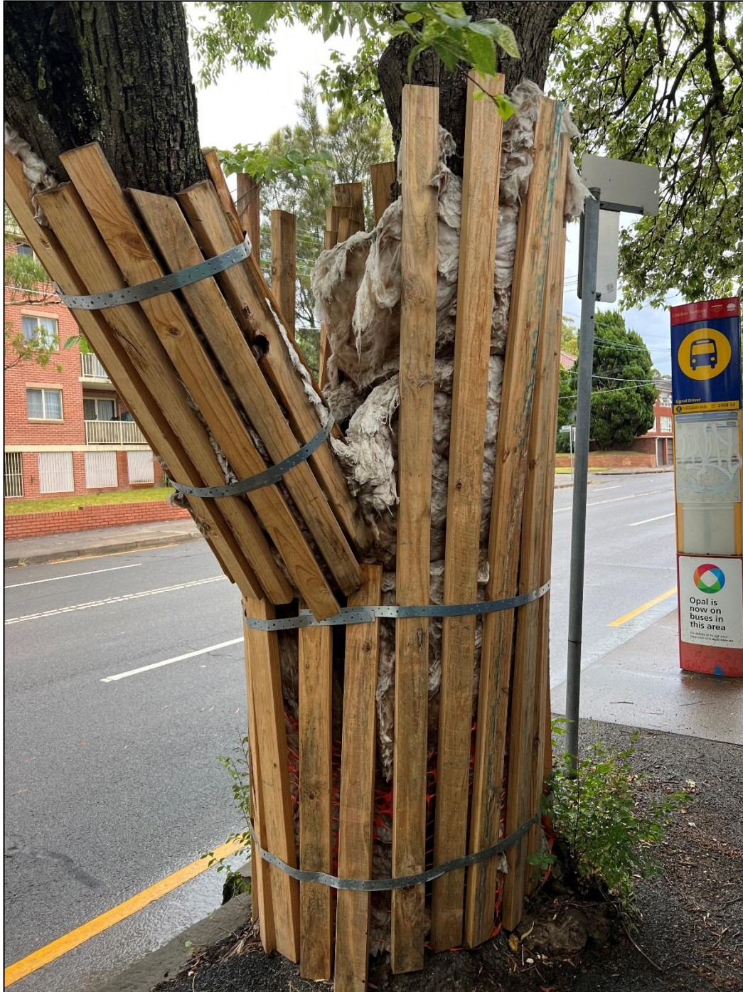
Figure 13. Trunk protection measures correctly installed in compliance with Sections 4.5.2 of AS4970 (2009).
