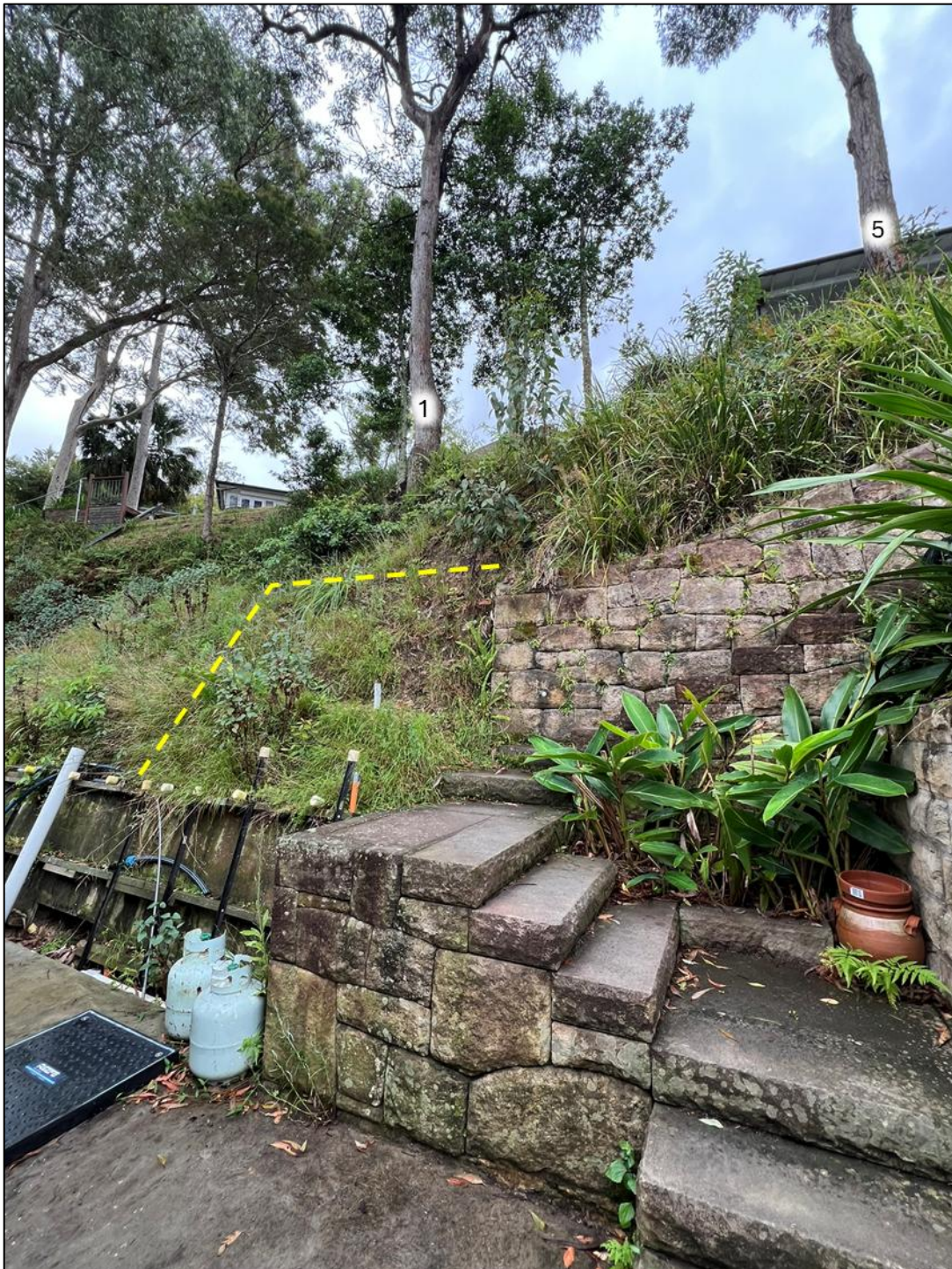
Figure 9. Existing slope, retaining wall and stairway will mitigate the impact of excavation required for the southern landing on Trees 1 and 5
