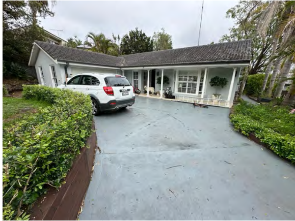
Photo 1: Frontage of the dwelling facing west.
