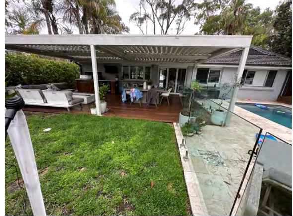
Photo 2: Rear of the dwelling facing south-east.
