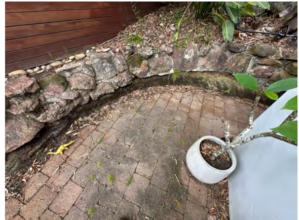
Photo 4: Inferred sandstone bedrock outcropping under stackrock landscaping wall.
