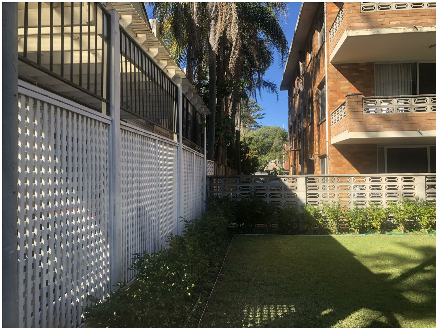
PHOTO 6 - BOUNDARY CONDITION BETWEEN PROPOSED BUILDING AND EXISTING NEIGHBOURING PROPERTY
