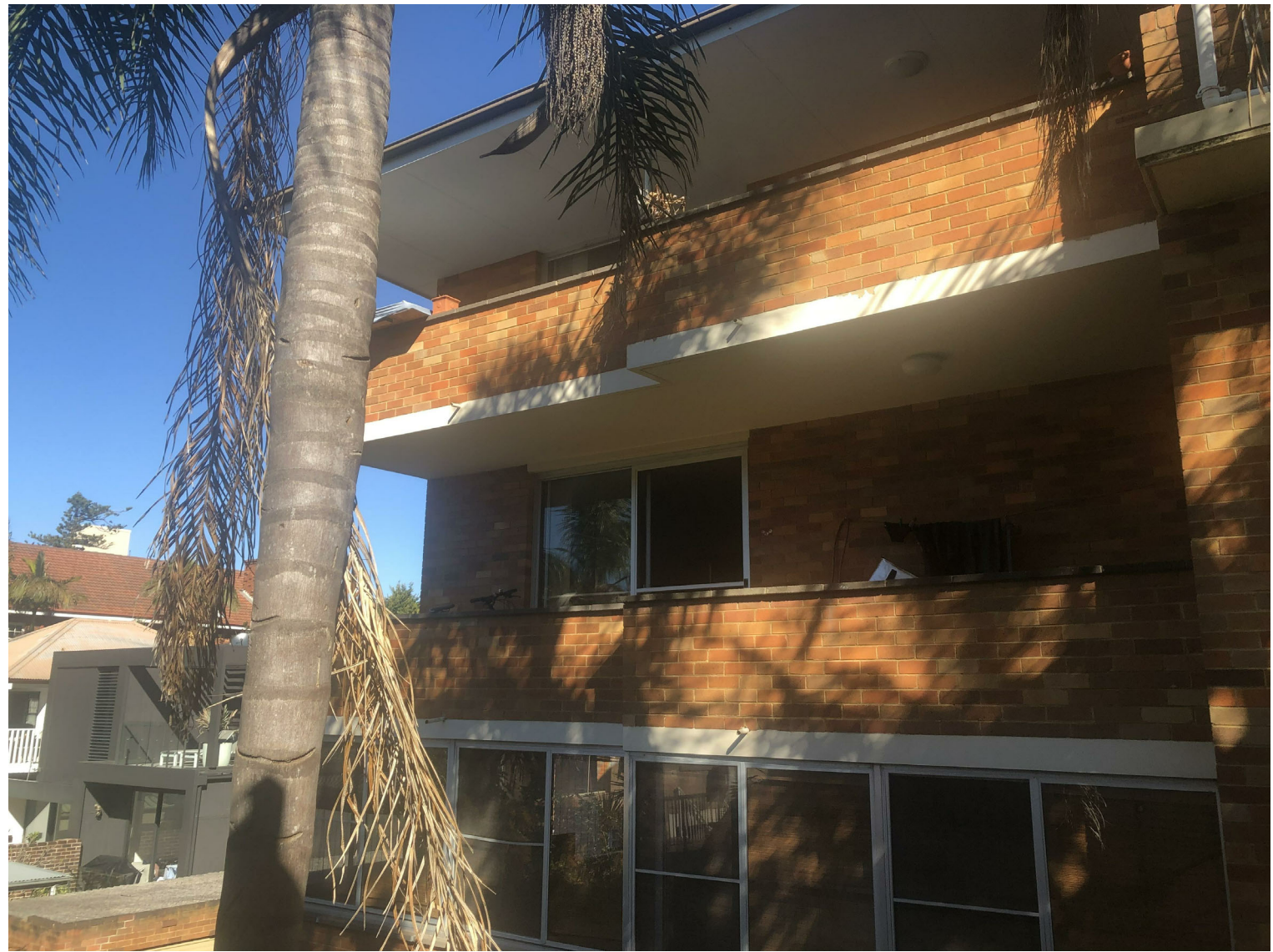
PHOTO 12 - BALCONIES OF NEIGHBOURING PROPERTY
