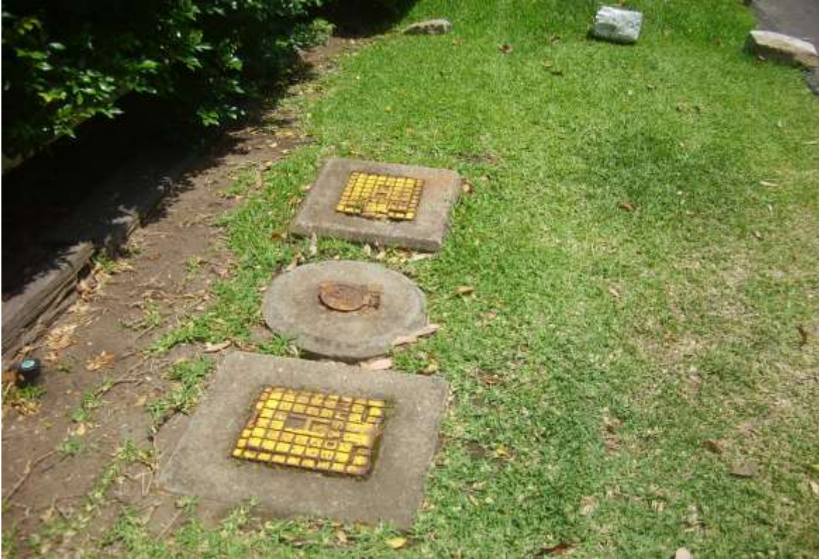
Photo 2 – Indicates the reticulated mains pressure fire hydrants located outside No.985 Barrenjoey Rd (Steve Brooks 2019).
