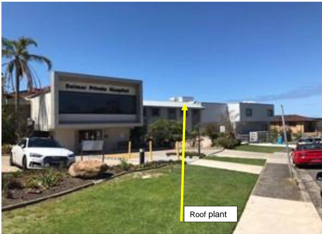
View from Quirk Street looking to the east. The roof plant is seen set back from the roof.
