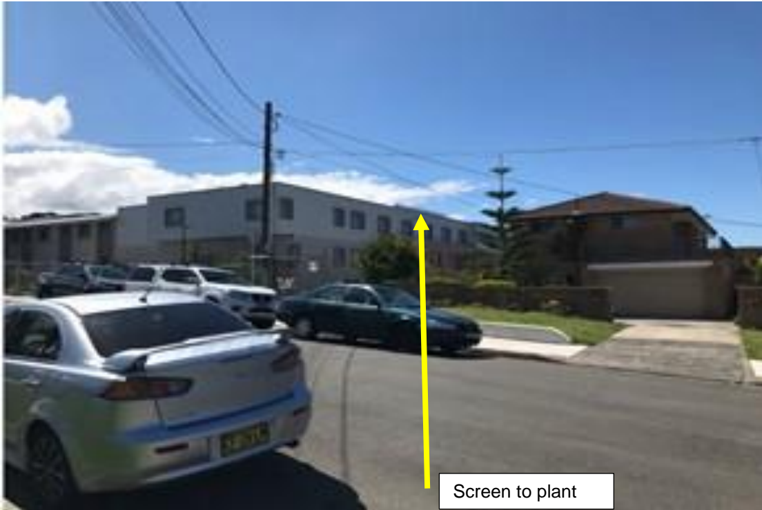
View from Quirk Street looking north-west. – photo taken with rooftop screen in place
