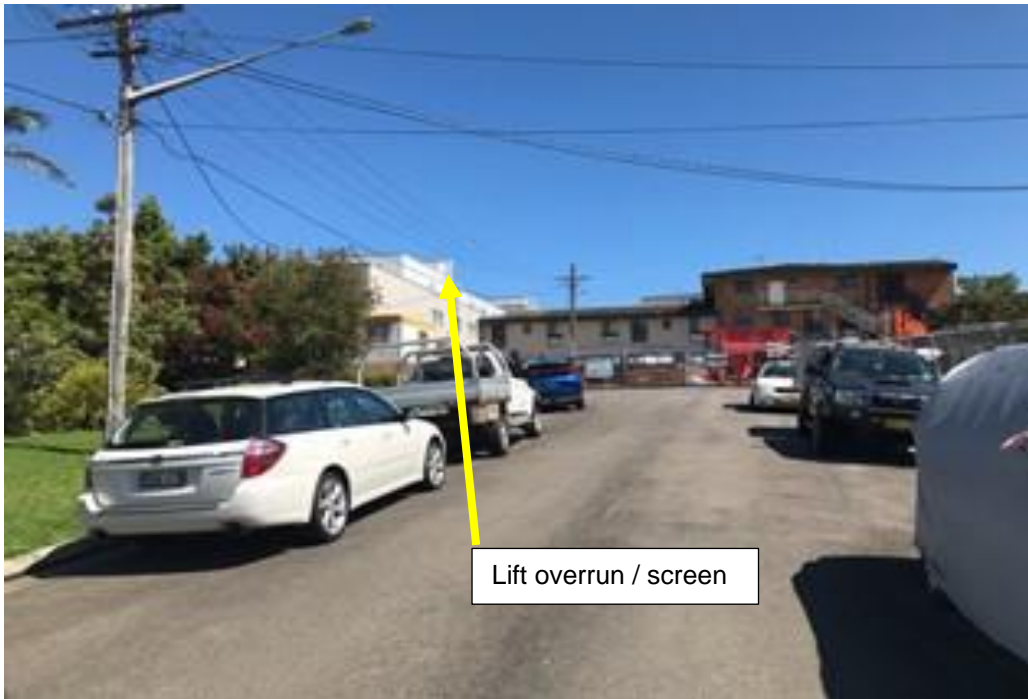
Views from Patey Street on approach from the north. The lift-over-run and screen can be seen in the distance.
