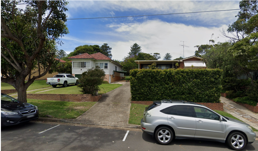
Figure 4 - View of properties No 7 & 8 viewed from Coronation Street
