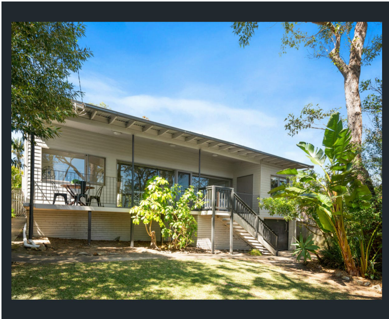
Figure 7- View of front façade existing residence 6 coronation st (source: LJ Hooker)
