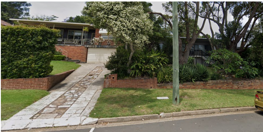
Figure 3 - View of properties No 7 viewed from Coronation Street
