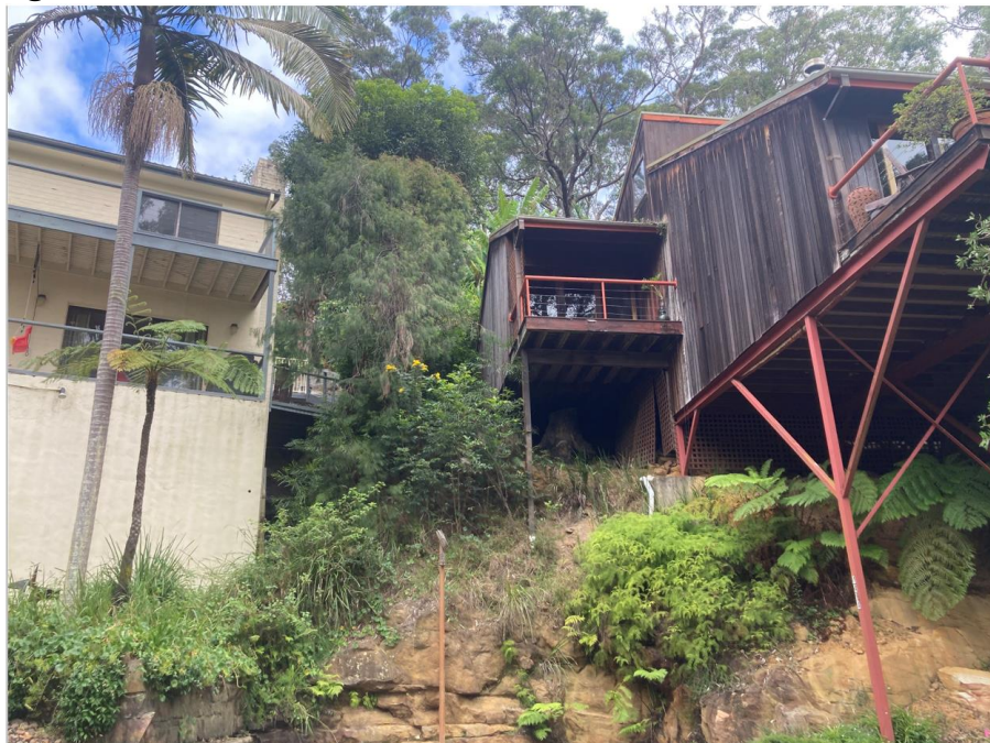
Figure 3: Eastern Elevation of 149A McCarrs Creek Rd
