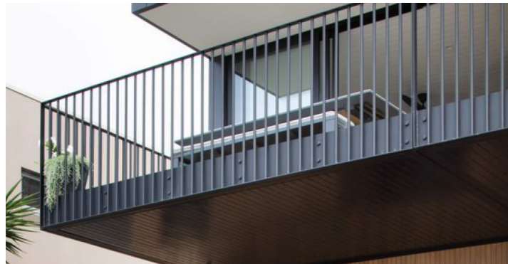
1 - STEEL BALUSTRADE POWDERCOAT FINISH 'BLACK' OR SIMILAR
