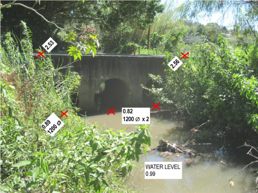
ID10-Culvert Sth us
