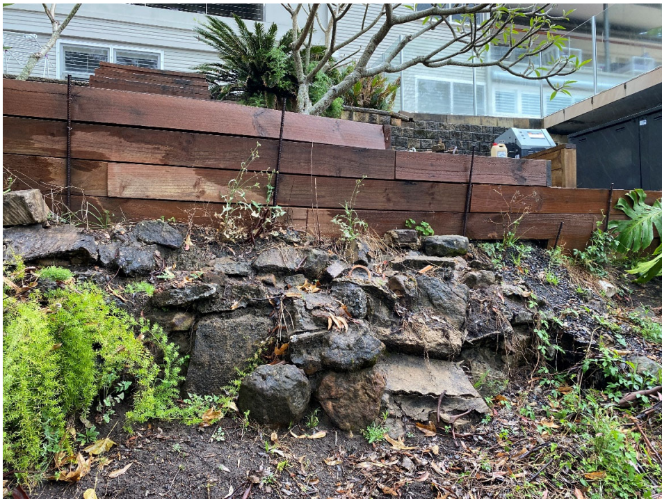
Image 5. Existing retaining walls to be replaced.
