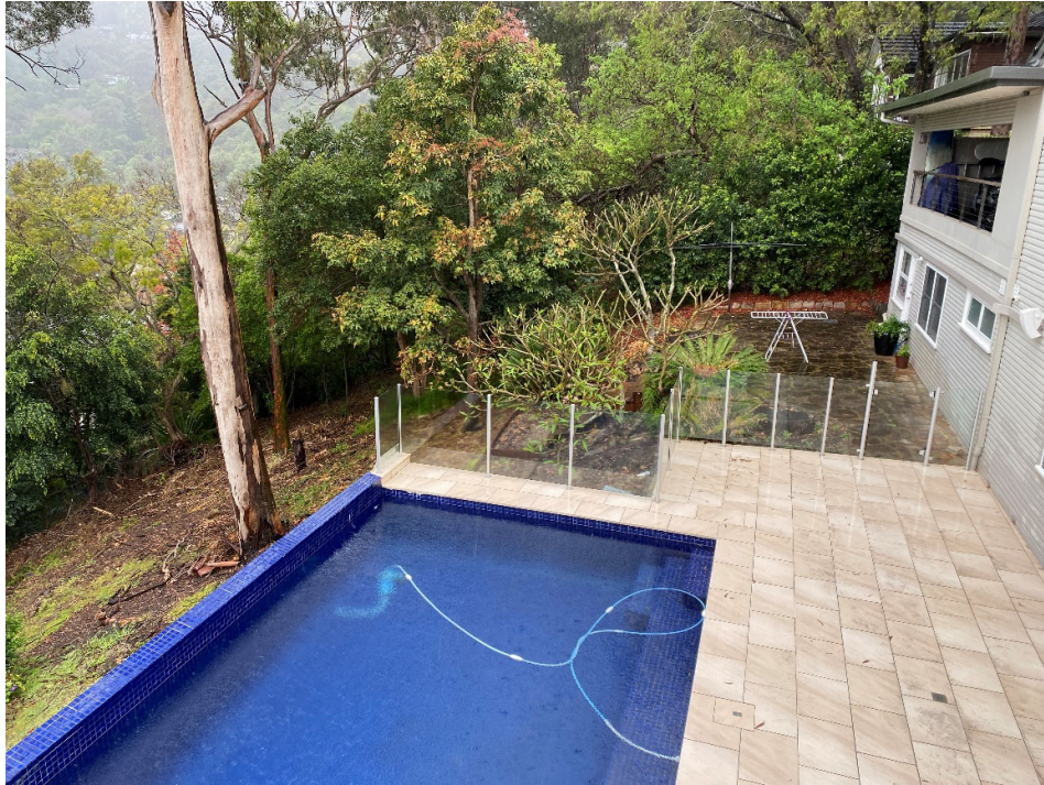
Image 2. Existing tiles and pavers to be replaced seen beyond the swimming pool. The protected tree to be removed can be seen to the left of the image.
