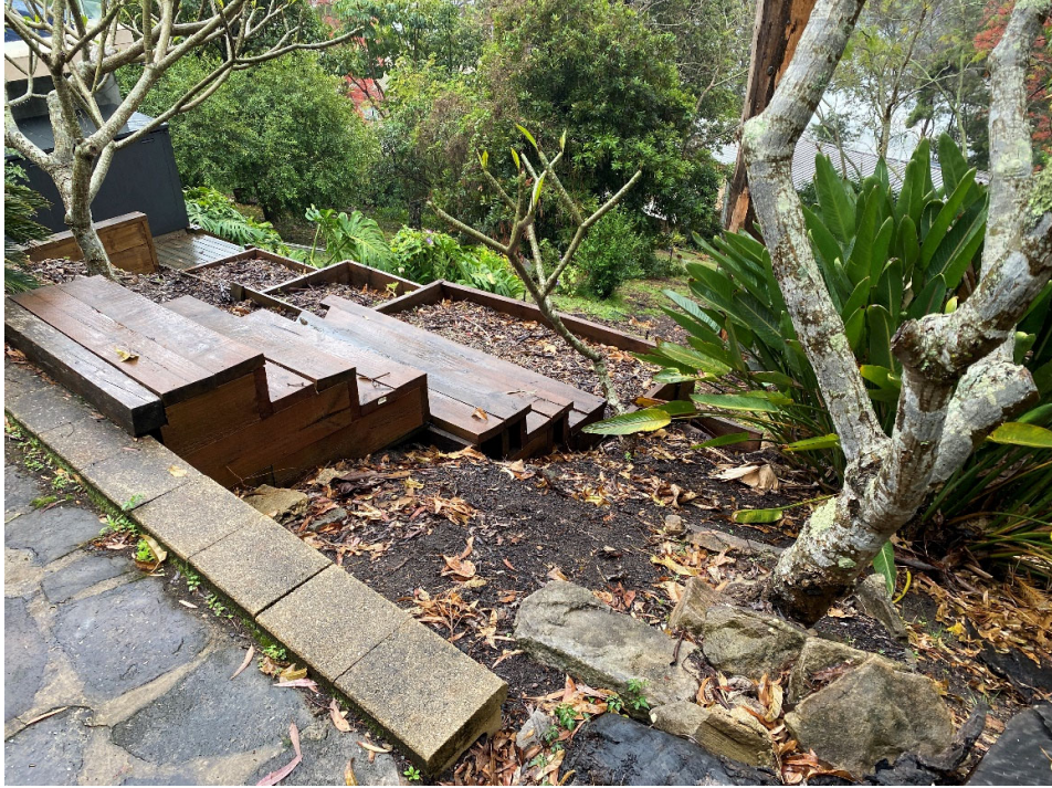
Image 4. Existing stairs and retaining walls to be replaced.
