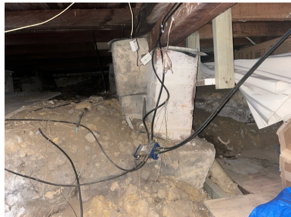
Photo 4: Cracked and sunken piers under the northern side of the house
