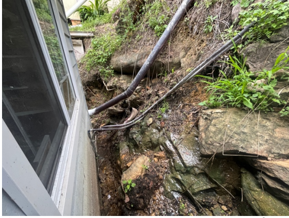
Photo 5: Bedrock at the southern rear corner of the dwelling, significant seepage
