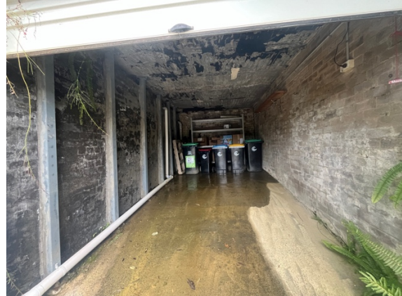
Photo 2: Brick garage, note left hand side wall is budging and has been braced by installation of vertical steel beams
