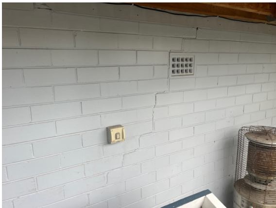
Photo 3: Cracking through the brick wall of the residence frontage, indicative of settlement of the northern corner of the house
