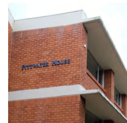
Face brick walls Painted concrete
