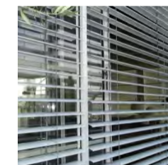
LO-1 External Louvres - Adjustable Powdercoat White
