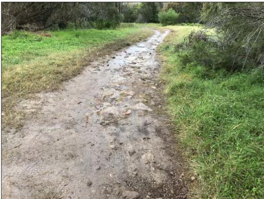
Photograph 4: Access track via Kirkwood Street, fill evident (builders rubble).
