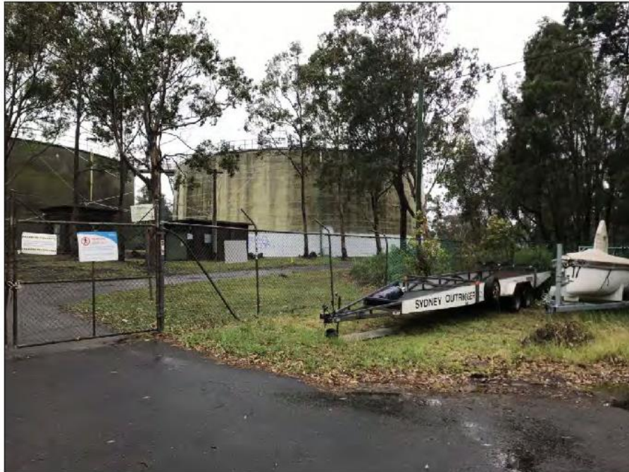
Photograph 1: Sydney Water Reservoir Site, Kirkwood Street.
