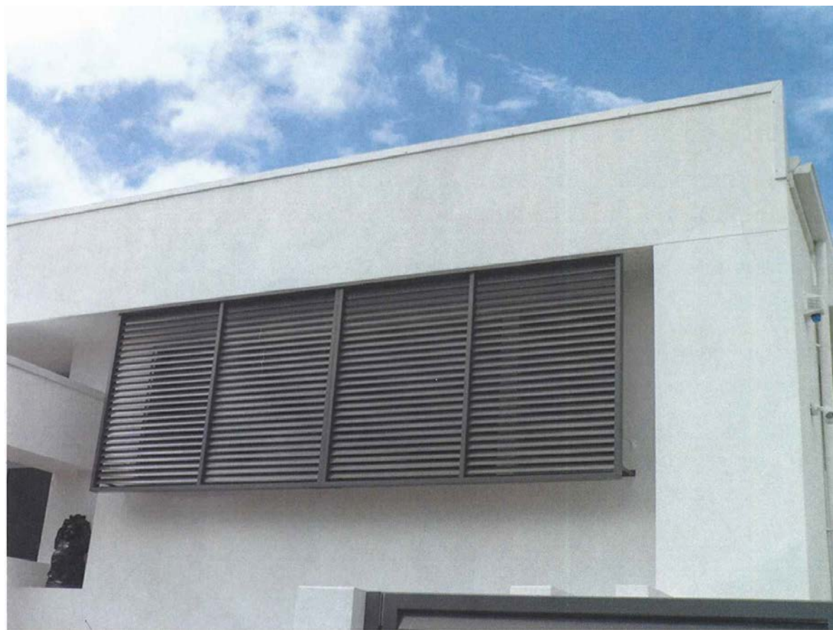
PROPOSED SCREENS *FIXED HORIZONTAL EXTERNAL LOUVRES - MINIMUM WIDHT OF 100mm AND MAXIMUM SPACING OF 100mm
