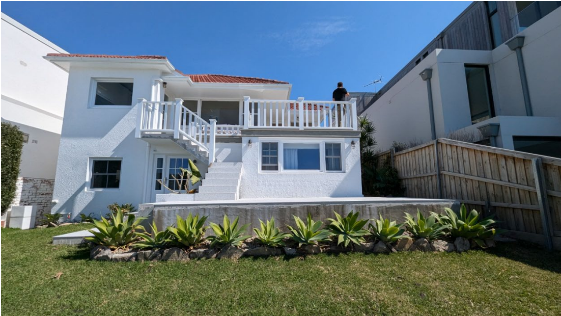
Subject site, 11 Loch St, as viewed from middle back yard looking west
