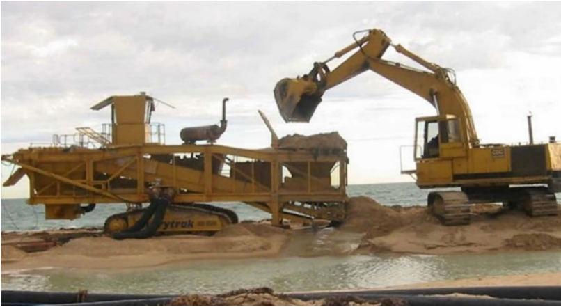
Slurrytrak system operating at Dawesville and Mandurah Inlets, Western Australia
