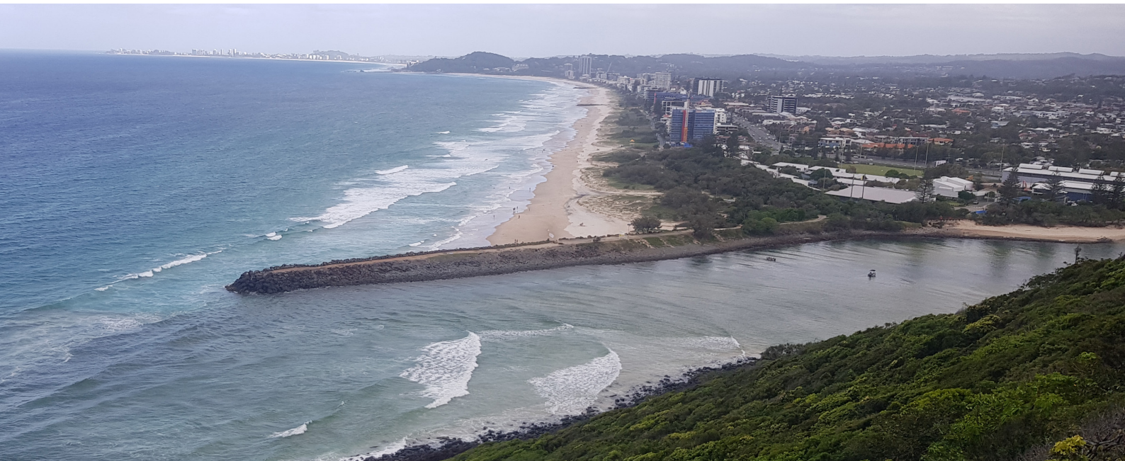
Example rock training wall at Tallebudgera Creek entrance
